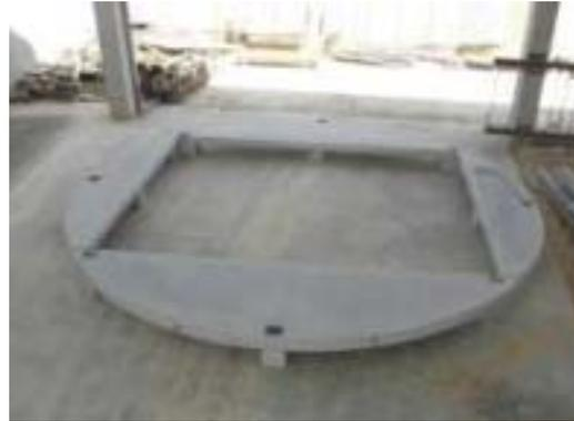
Manufacturing process of these four elements, the semicircular slabs are designed in two pairs of two different sizes, the largest weighing 4175 kg each and two smaller 2300 Kg.
